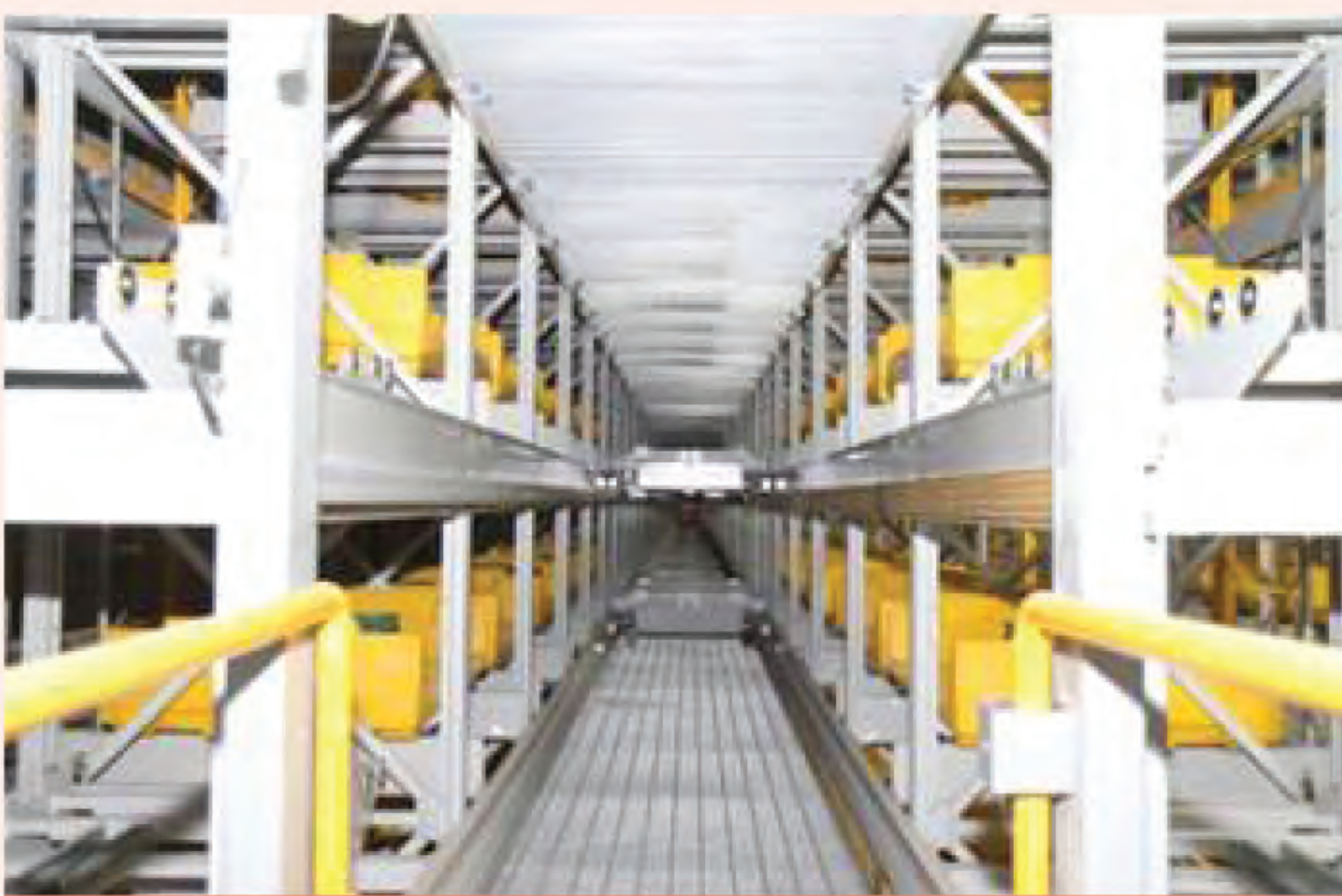
Early baggage storage system
