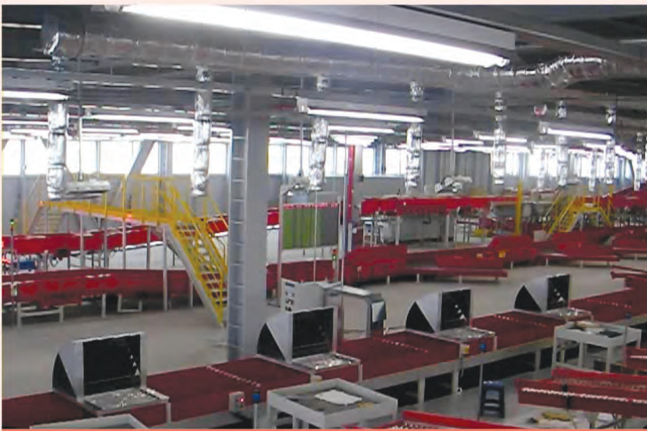
DHL Distribution Center
