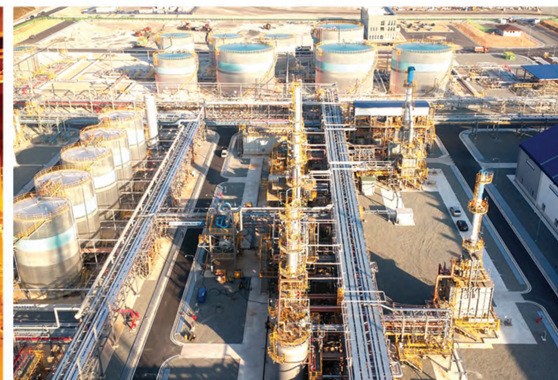
Construction of a needle coke plant
