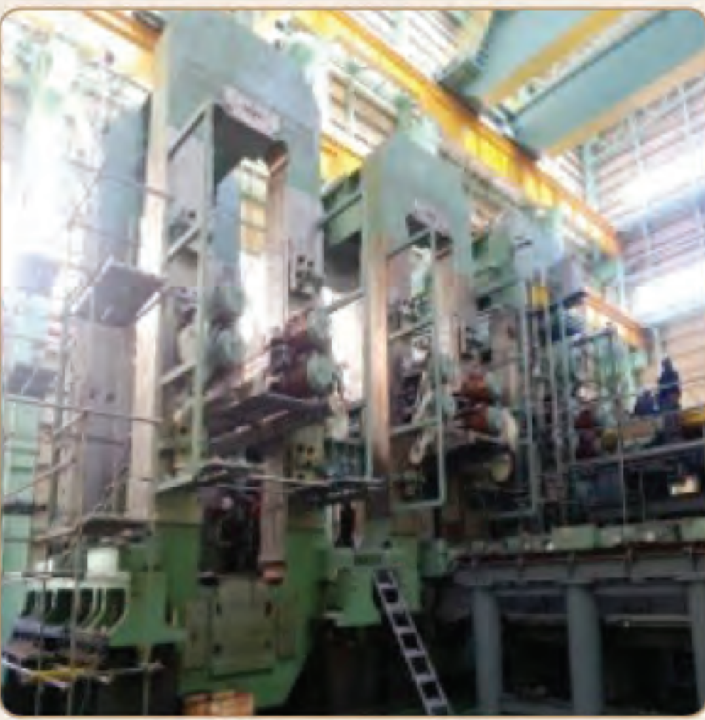
Assembly of a rolling mill
