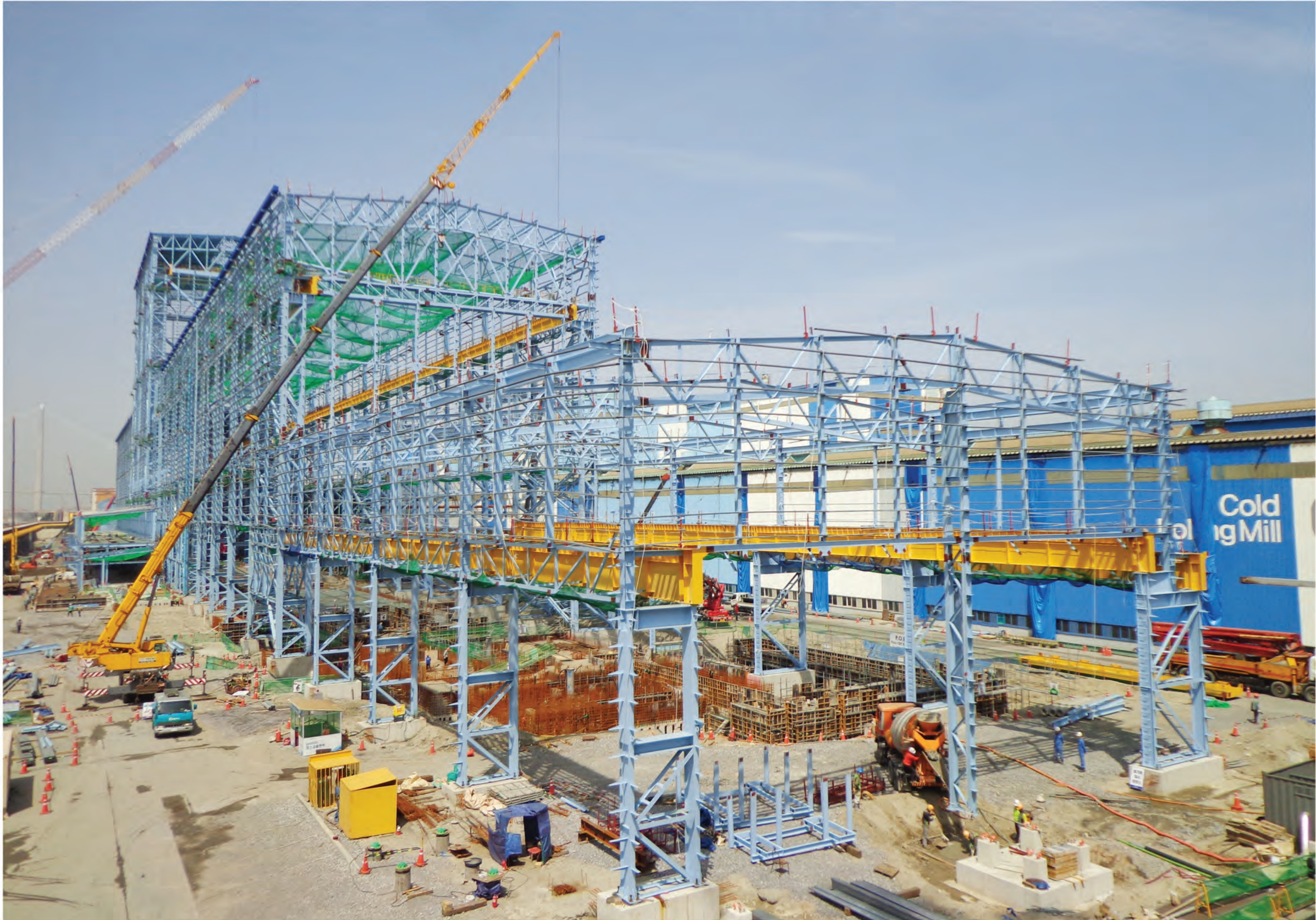
A project of constructing 7CGL at the Gwangyang Iron Mill
