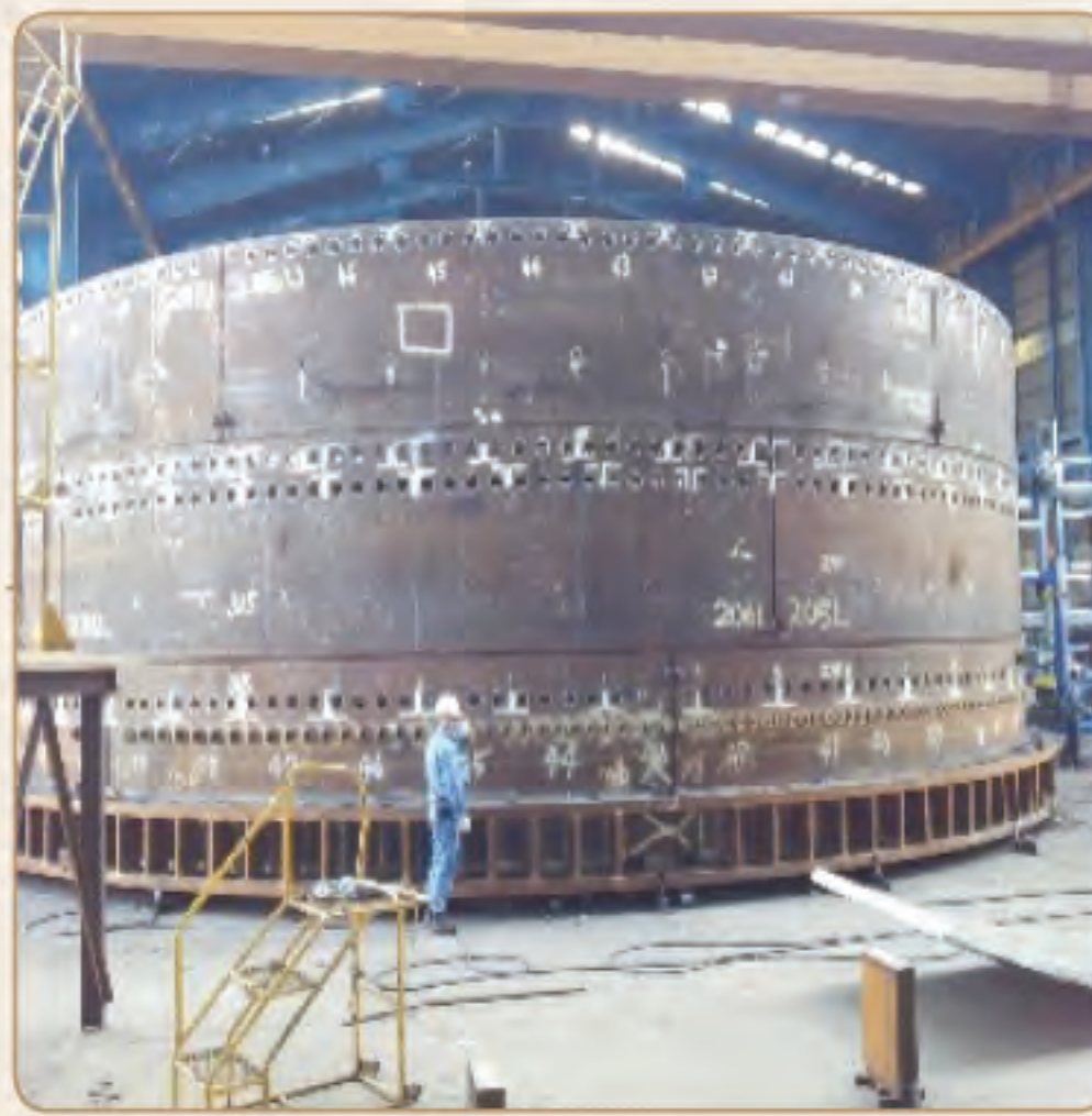
Temporary assembly of Finex 2 million tons in Pohang
