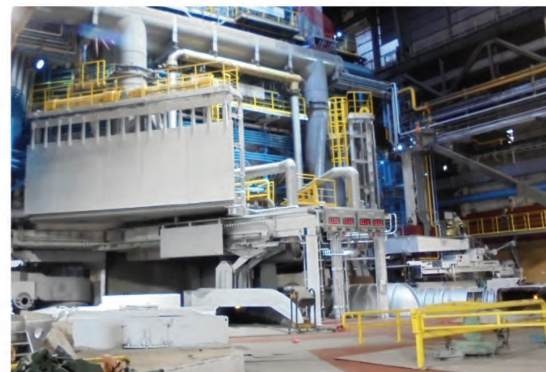
3 Blast Furnace at the Pohang Iron & Steel Mill 주상설비
